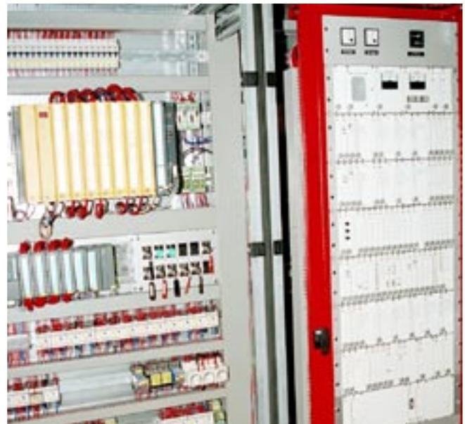
A view inside the control panel. Left, the fail safe PLC (yellow) and the Remote Supervision System rack on the right.
