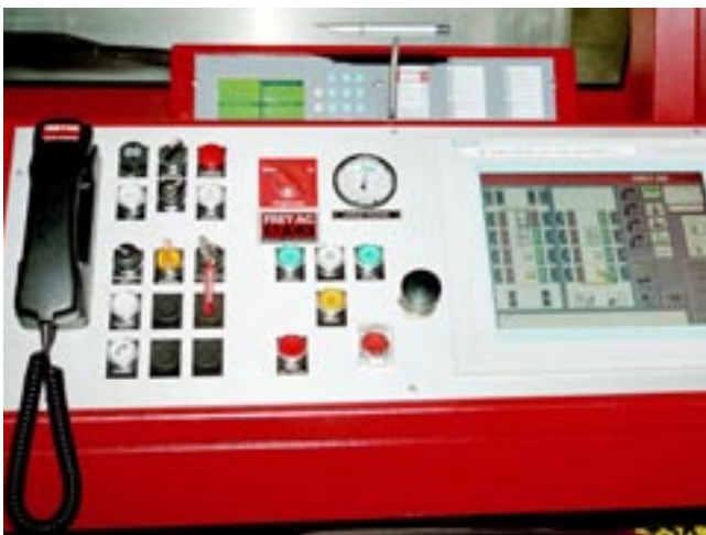
Control station with touch panel in the upper drivers compartment.
