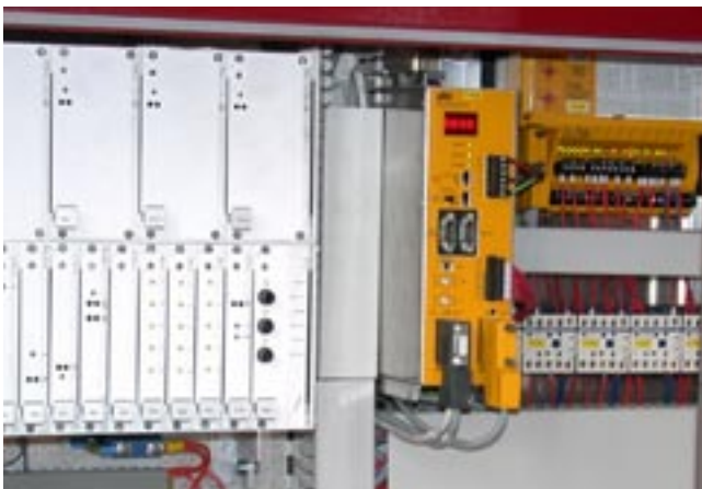
ASafety Bus system allows processing of all 140 safety functions in the car.
